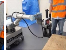
HRT for Installing Screws
